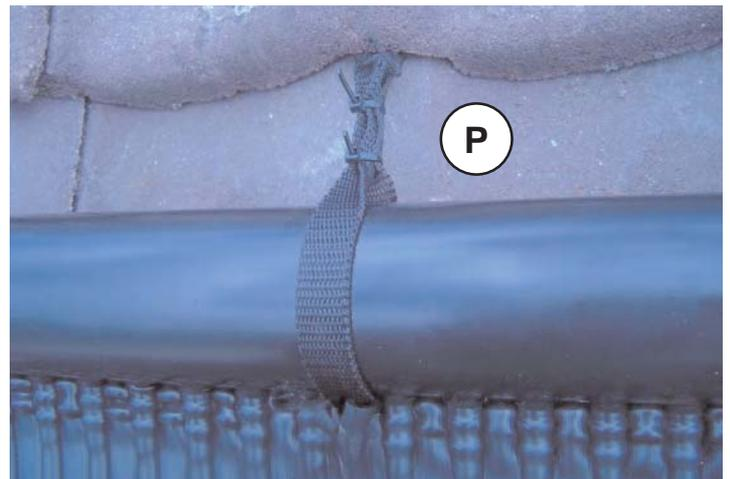
Nylon strapping can also be used (horizontally) across the width of matting to secure it to the roof structure (Q). Place straps 1 metre apart.
