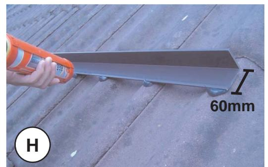
Note: the adhesive is only as good as the surface it is applied to, therefore ensure the surface is free of any loose foreign material.
