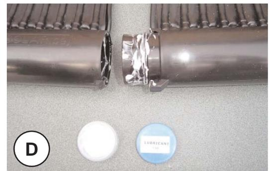
**STEP 3** Push the rubber edges (E) together so the absorbers (EPDM matting) are united as a whole.
