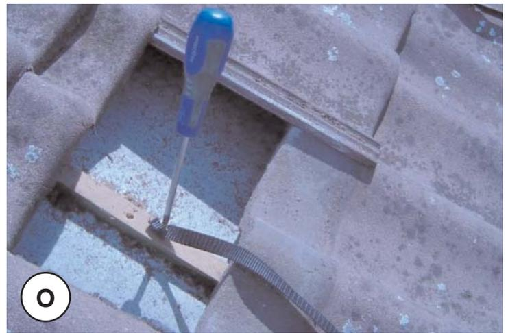
Fix 50 cm long nylon strips on the roof support batten every 66 cm as per step 7 on page 6. Afterwards put the roof tiles back in place so the nylon strips stick out 30 cm. Attach the nylon strips that stick out of the roof around the collector. Attach 2 tie-wraps to every nylon strip.
